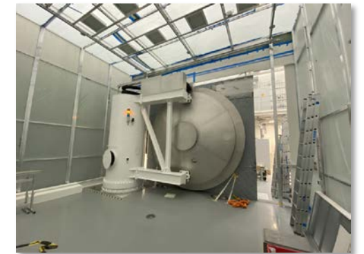
cleaning & leak check
